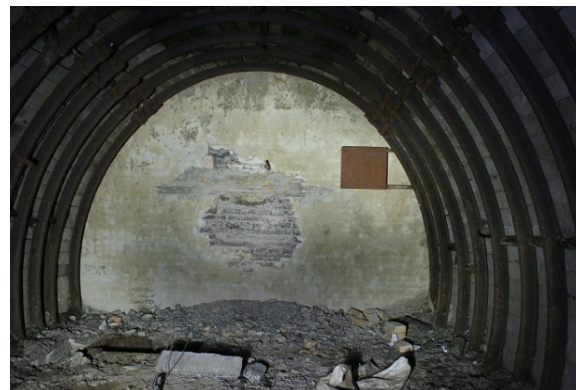
Fig. 1 View of the underground gallery
